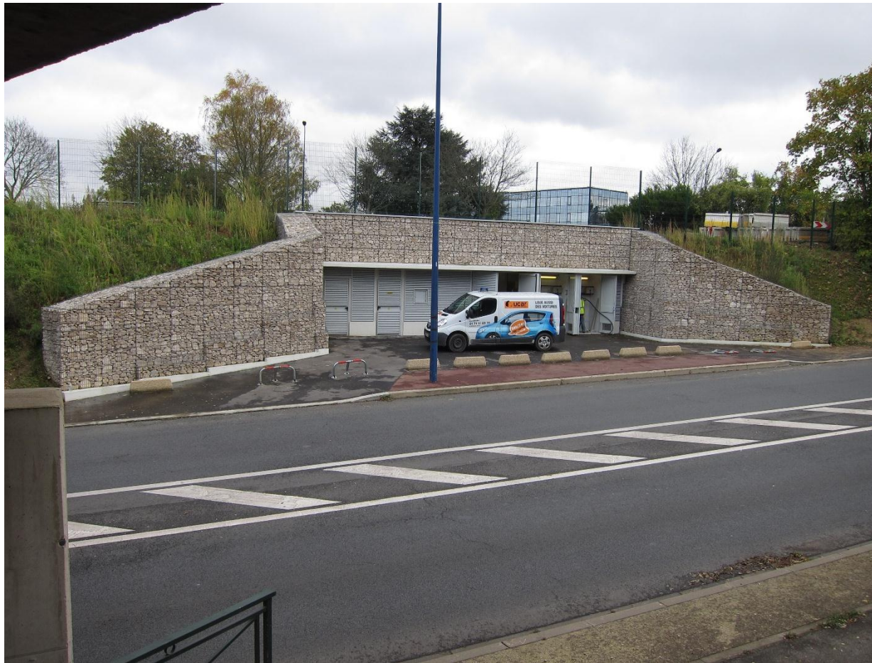
Illustration 4. Mur en gabion, source SARA
